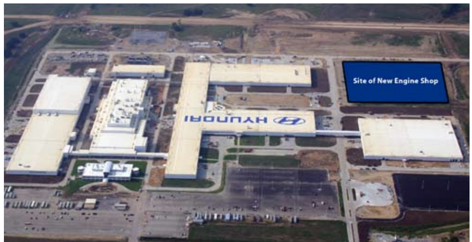
This aerial view of HMMA shows the location of the new Engine Shop which is under construction.
